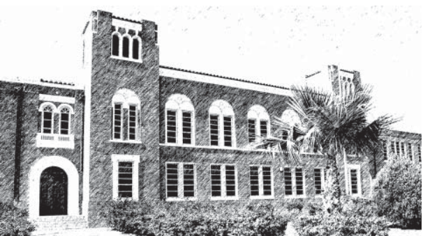
The new BISD Museum and James R. Murphy Center are located in the Central Administrative Building Complex on Palm Boulevard.
